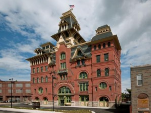
American Brewery Building, Baltimore MD
