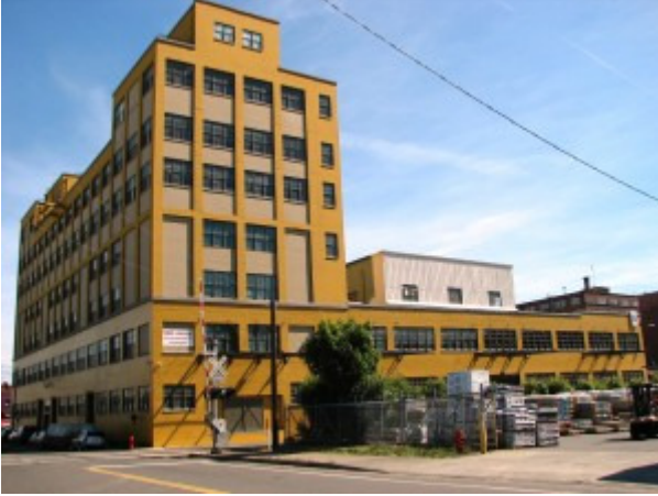
B&O Warehouse, Portland OR
